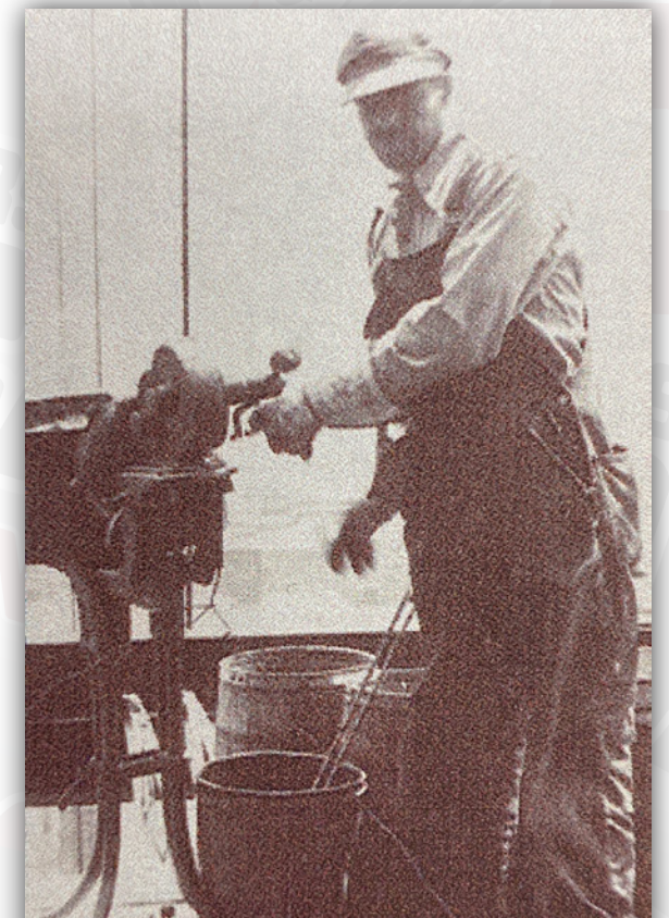
Local 99 member Frank Bill works on a five-story addition to the State Farm Insurance Building corporate headquarters in downtown Bloomington in June 1934.
