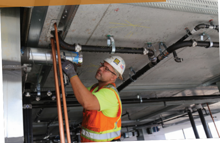
Local 78 Brother Eli Houta installs plumbing at the Metropolis Residential Tower 3 in 2017.
