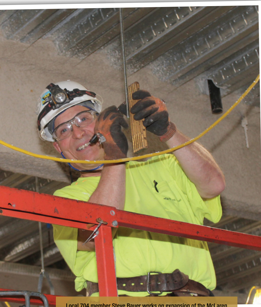
Local 704 member Steve Bauer works on expansion of the McLaren Macomb Hospital in 2019 on the day before he would retire after 41 years as a member of the local. (Courtesy of The Building Tradesman.)
