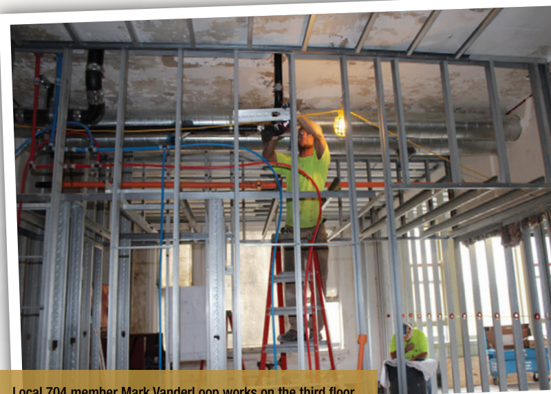
Local 704 member Mark VanderLoop works on the third floor of the then-98-year-old David Whitney Building in Detroit during its renovation in 2013 to create retail space, a boutique hotel and apartments. (Courtesy of The Building Tradesman.)
