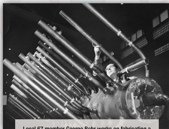
Local 67 member George Behr works on fabricating a pipe header for a nuclear power plant while working at Crane Piping during the 1960s.
