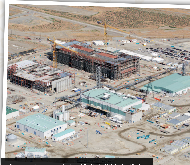
Aerial view of ongoing construction of the Hanford Vitrification Plant in 2017. (Photo Credit: Bechtel National, Inc.)
