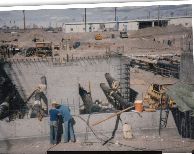
Construction of the Tank Farm in the 200-E area of the Hanford Site with Local 598 members in 1985.
