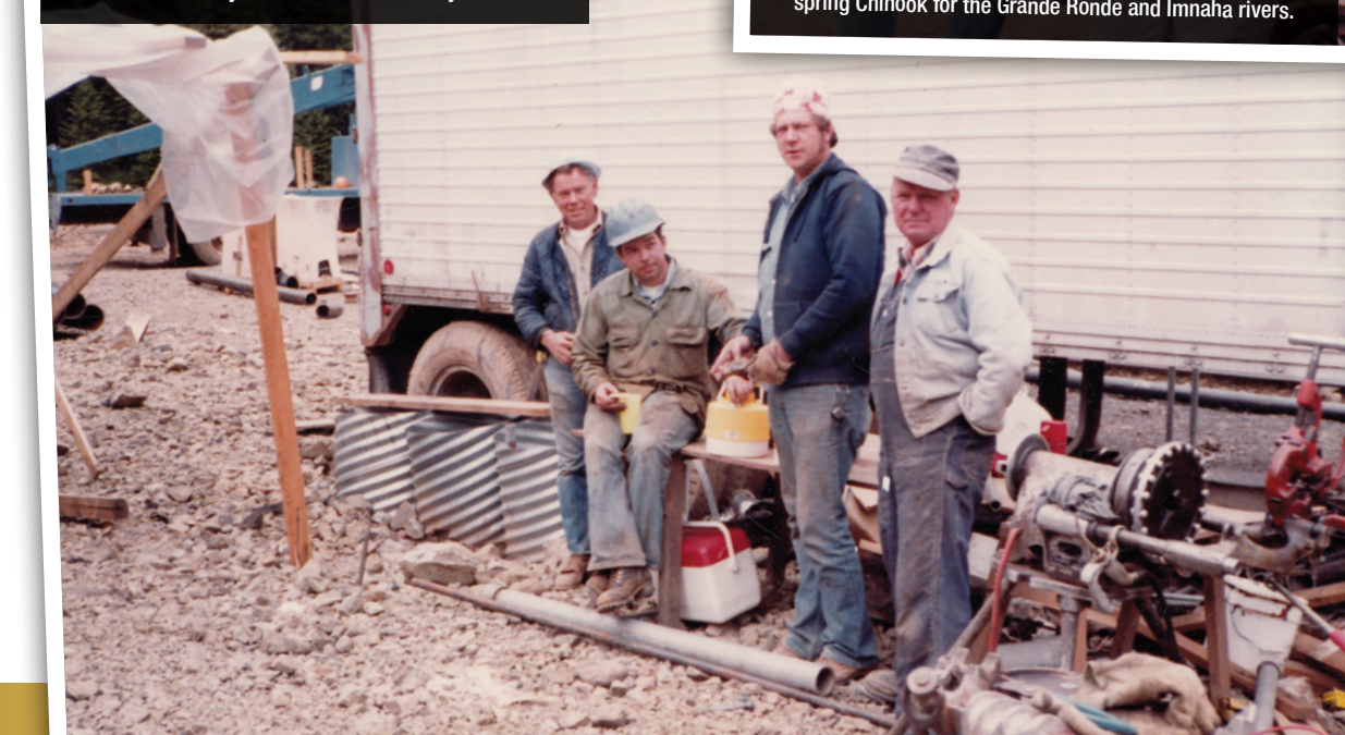
Local 598 members (left to right) Dale Dubin, unknown, Roger Hadden and Don Johnson at the Lookingglass Fish Hatchery construction site in May 1981.
