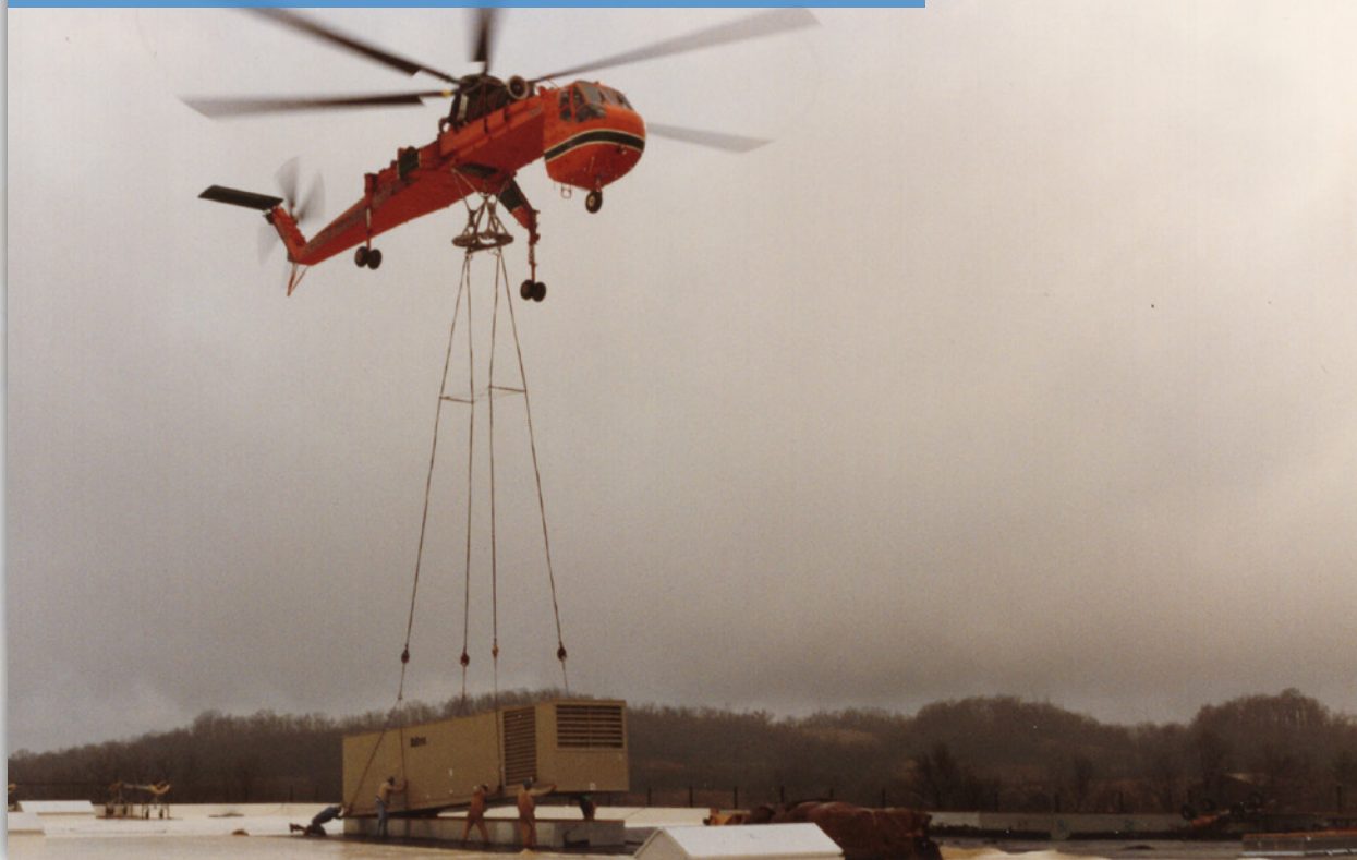
Local 572 set air-control units on top of the new GM Saturn plant being built in Nashville in 1990.
