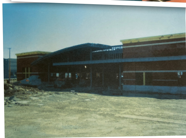
The new (and current) Sprinklerfitters Local 268 Union Hall and Training Center at 1544 South Third in South St. Louis under construction in 2005 before the local moved into the facility late that year.
