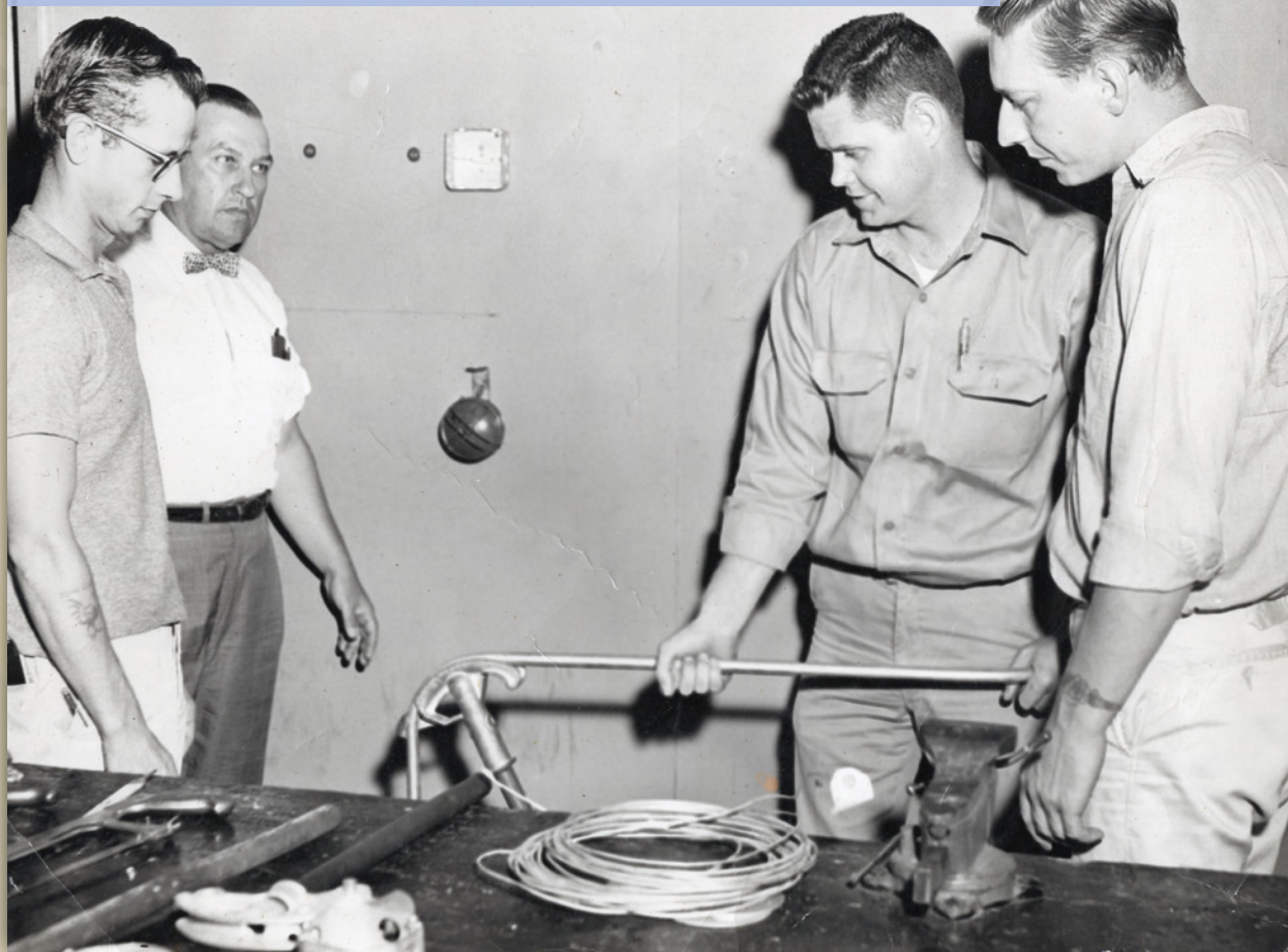
Local 268 sprinklerfitting training instructor Joe Karl (center) and apprentices (right) John O'Donnell and Gordon Lundak Sr. (a future Local 268 business manager) are joined by an apprentice from Kansas City at a St. Louis Automatic Sprinkler Industry Joint Apprenticeship Committee training class sometime during the 1950s.
