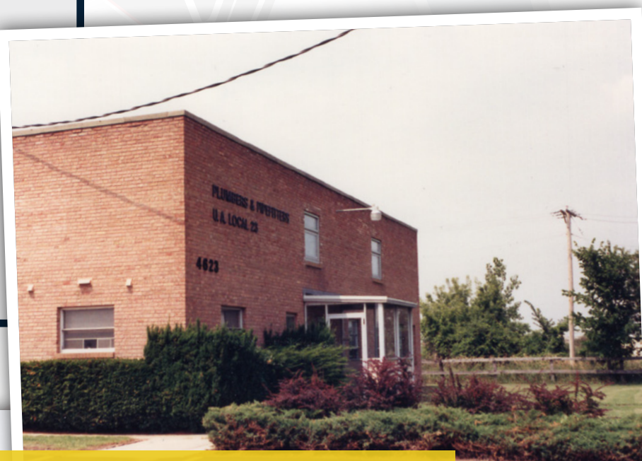
Local 23 Union Hall and Training Center at 4623 Boeing Drive in Rockford.
