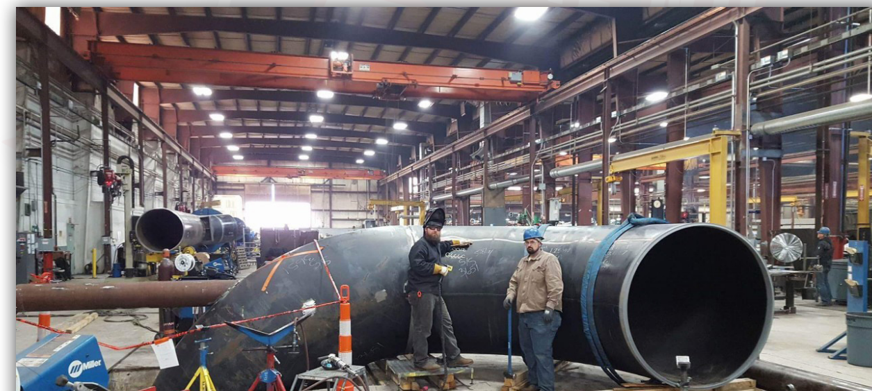
Current Local 140 Business Agent/Vice-President/Organizer Cody Weaver (left) and Local 140 member Jeff Hurst work on welding a 68-inch, 1.25-inch-thick pipe in the CB&I fabrication shop in Clearfield, Utah, in January 2017, after which it would be sent to a liquefied natural gas plant in Texas. Brother Weaver was a third-generation member of the U.A. to work in the shop, as his grandfather, Lavar Weaver, ran it at one time and his father, Steve Weaver, and uncle, Clair Weaver, also worked in the shop for many years.
