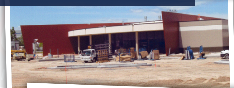
Local 140 and its members build the new Utah Career Center in 2010, which since opening in November of that year has provided vocational training to the state's U.A. piping apprentices and members.
