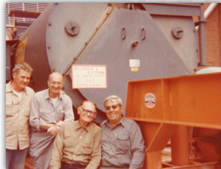
Local 101 members (left to right) Mack Carl, Bud Kiefer, Business Manager William K. Adrian and Roy Kopf break during a job installing a boiler at the Military Airlift Command Building at Scott Air Force Base sometime during the 1970s.
