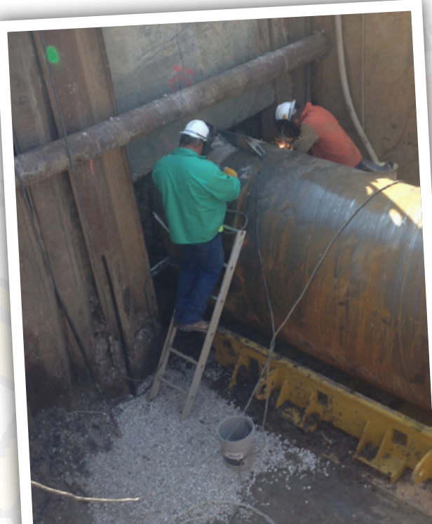
Local 101 members Lucas Mense and Jon Schwartz weld a bore casing under Illinois State Route 159 and Route 15 while working on the City of Belleville sewer-main extension project in 2016.
