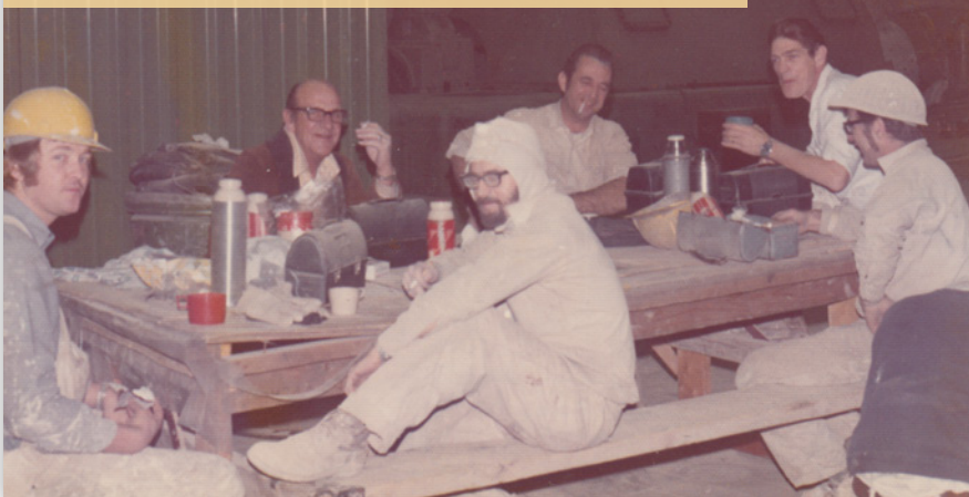
Local 845 members Bob Stayland, Roy Jones, Dick Hoisington, Dave Murphy, Bill Ballont and Pete Simmons working at the Lansing Power Station plant in January 1973.
