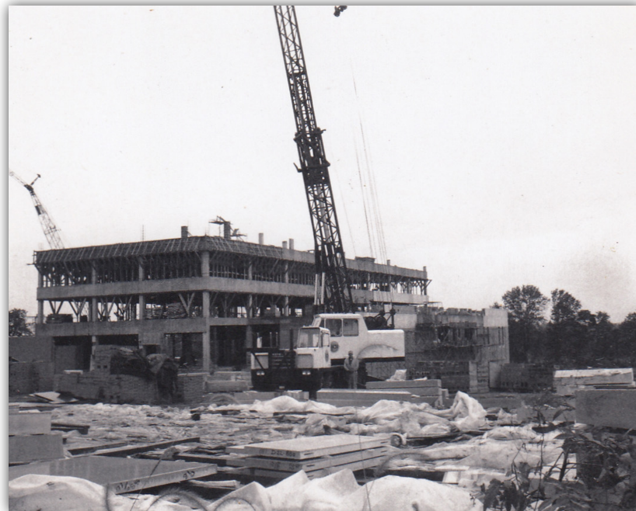
Local 841 member Brother Ike Wilkinson operates a tower crane during construction of the new Greene County General Hospital in Linton, Indiana, in October 1971. The hospital opened in April 1974.
