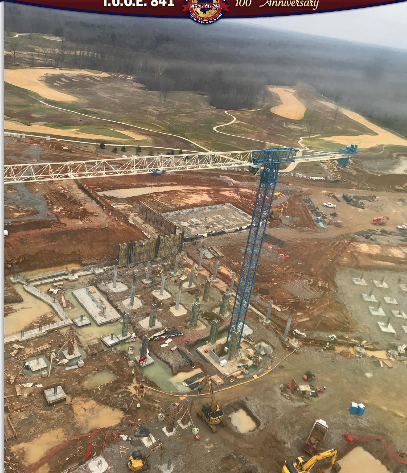
Local 841 members work on construction of the new Indiana University Health Bloomington Hospital in April 2019 for its scheduled opening in late 2021.
