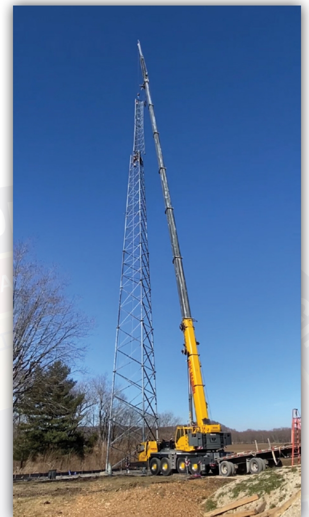
A Local 841 crew removes a cell tower near Martinsville, Indiana, in March 2021 to make way for construction of Interstate 69 through the area.
