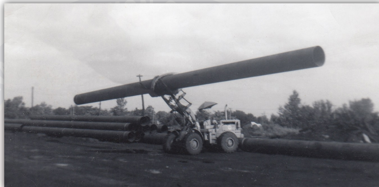
Local 841 member Brother Pud Saunders moves an 80-foot-long, 24-inch pipe on a job in Mattoon, Illinois, sometime during the early- or mid-1960s.
