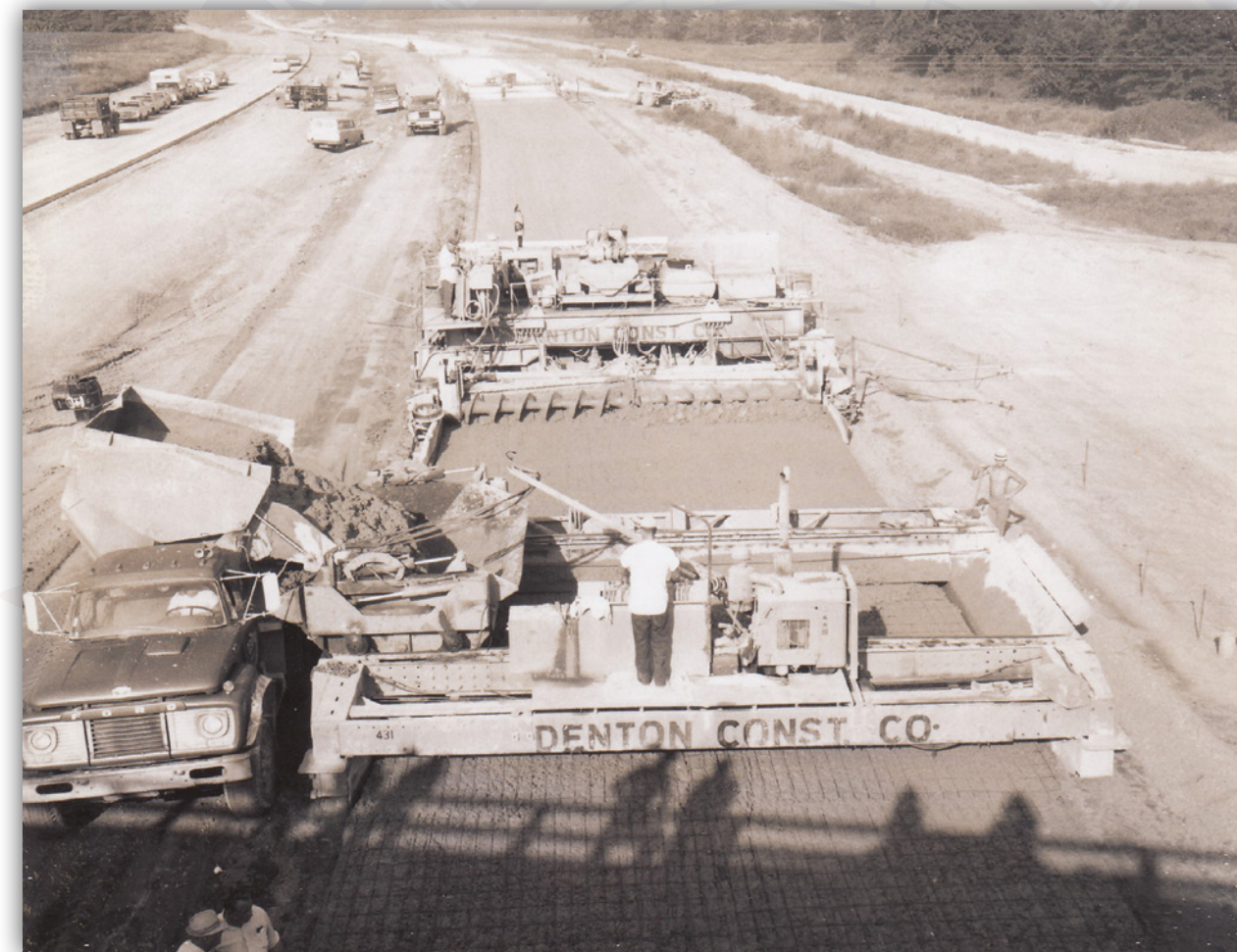
Local 841 members working for Denton Construction Company build a segment of the new Interstate-70 highway beneath the Harmony Road (now North County Road 200 East) overpass southeast of Brazil, Indiana, in August 1968
