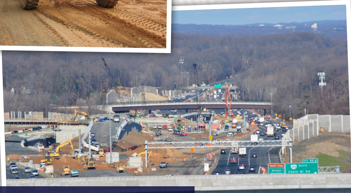
Local 77 operating engineers install High Occupancy Toll (HOT) express lanes on Interstate-495 around Washington D.C. and Northern Virginia in 2009.
