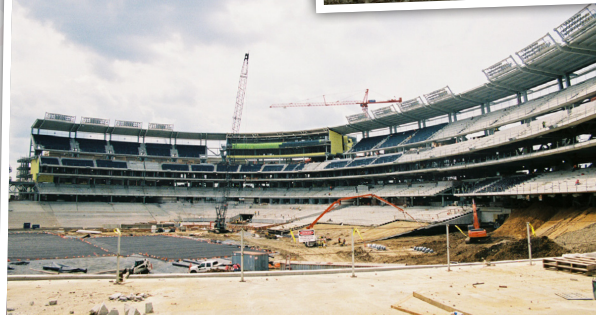
Local 77 operating engineers work on construction of the new Nationals Park baseball stadium along the Anacostia River in the Navy Yard neighborhood of D.C. from 2006 into 2008.
