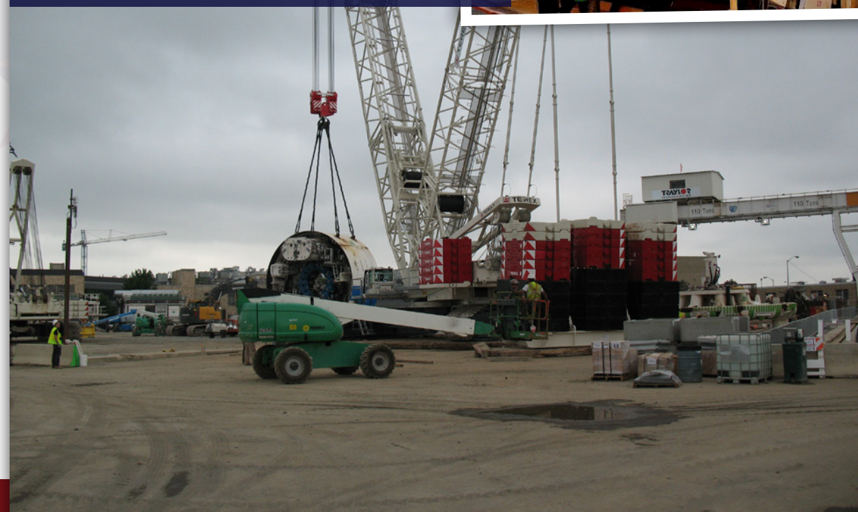
Local 77 operating engineers work on construction of the Blue Plains Tunnel, a 4.5-mile combined sewer overflow tunnel for DC Water’s Clean Rivers Project, in 2013.
