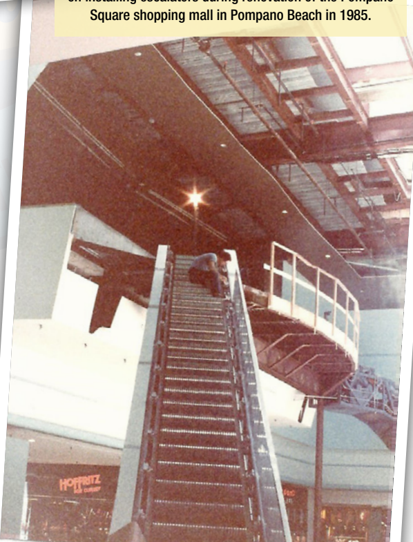
Local 71 members William Grubb (top photo) and Charlie Reeder (left, middle photo) and an unknown member work on installing escalators during renovation of the Pompano Square shopping mall in Pompano Beach in 1985.
