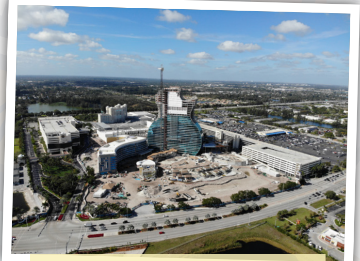
The Seminole Hard Rock Cafe and Resort in Hollywood, Florida, under construction with Local 71 members in December 2018. (Photo from Wikimedia Commons user Yanjipy.)
