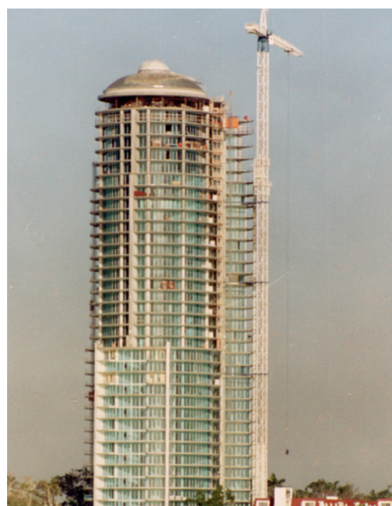
The 40-story Bristol Tower condominium high-rise in Miami under construction with Local 71 members in 1993 before it was completed and opened later that year.
