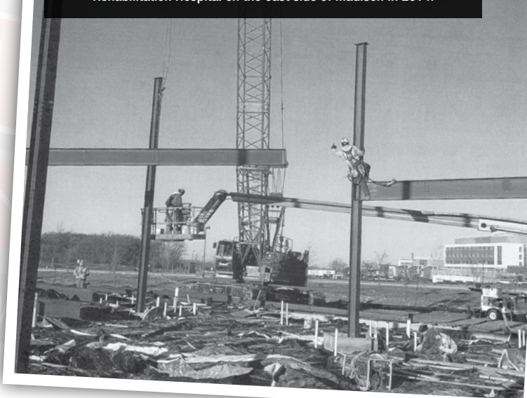
Local 383 iron workers (left to right) Brian Falleck, Jon Kinney and Jonah Getter erect the steel frame for the new UW Health Rehabilitation Hospital on the east side of Madison in 2014.
