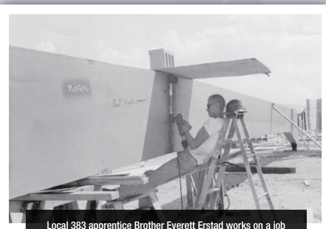
Local 383 apprentice Brother Everett Erstad works on a job while training as part of his apprenticeship in August 1959.
