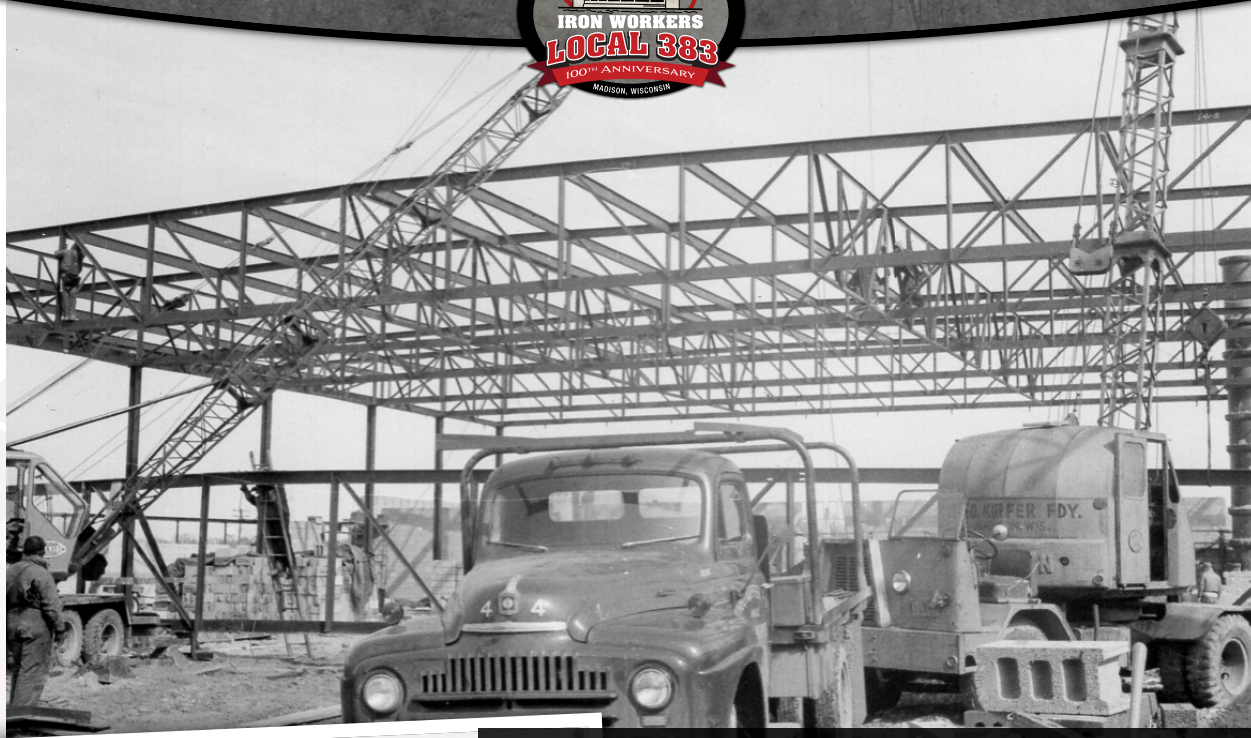
Local 383 members erect the original Monona Grove High School in Monona, Wisconsin, for its opening in 1955. (The school was replaced with a new building in 1999.)
