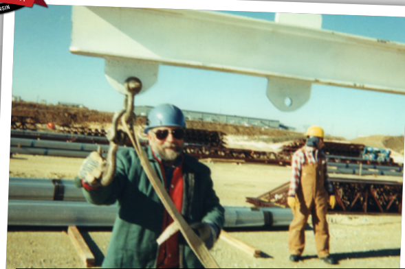
Local 383 members Brother Paul Fauerbach (left) and Brother Curtis Bell work on construction of a Sub-Zero and Wolf companies appliances warehouse in Madison in 2000.
