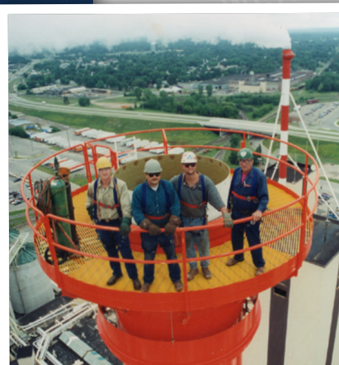
Local 383 members (left to right) Wayne Peplinski, Dennis Peplinski, Waylon Dupee and Foreman Gus Peplinski make up the connector and welding crew working on erection of a stack for the Verso Corporation's Kraft paper mill in Wisconsin Rapids in July 1996.
