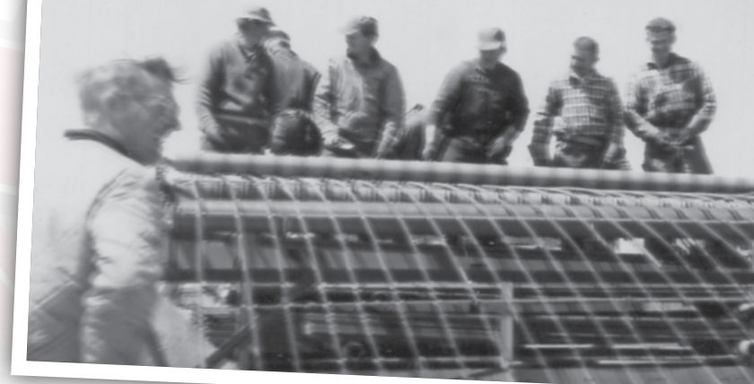
Local 383 members place reinforcing rebar for the construction of Interstate-90 through the local's jurisdiction in 1961.
