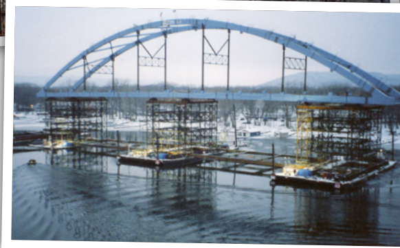
Local 383 iron workers erect the new Cameron Avenue Bridge over the Mississippi River between downtown La Crosse, Wisconsin, and Barron Island in 2004 for its opening the following year, when it and the existing Cass Street Bridge would make up the Mississippi River Bridge.
