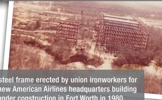
Local 263 and Local 481 members celebrate during the "topping out" party after the highest steel beam was put into place on the new American Airlines headquarters building being built in Fort Worth in 1980.
