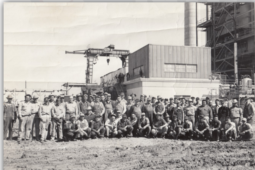
Local 72 crew that worked on construction of the Lake Creek Power Plant in Waco in 1953.
