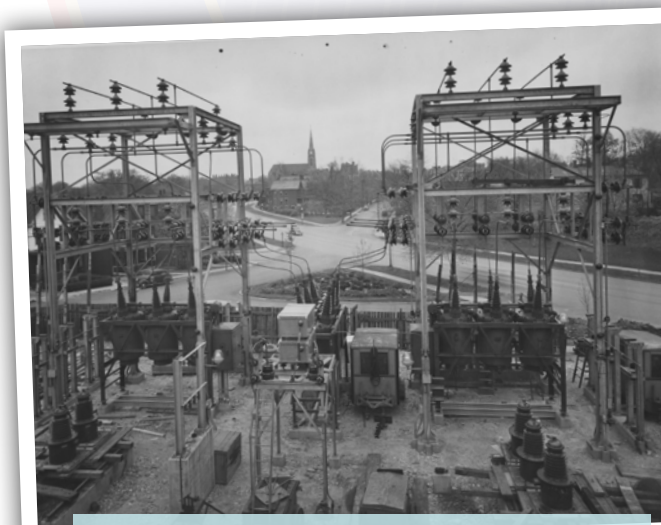
The Cincinnati Gas & Electric Company's Walnut Hills Substation 66-kilovolt switchyard in Cincinnati shown in April 1948.
