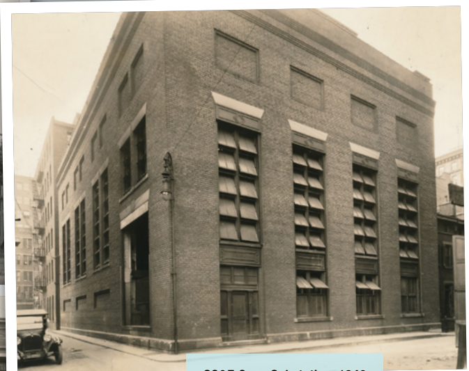
CG&E Gano Substation, 1940
