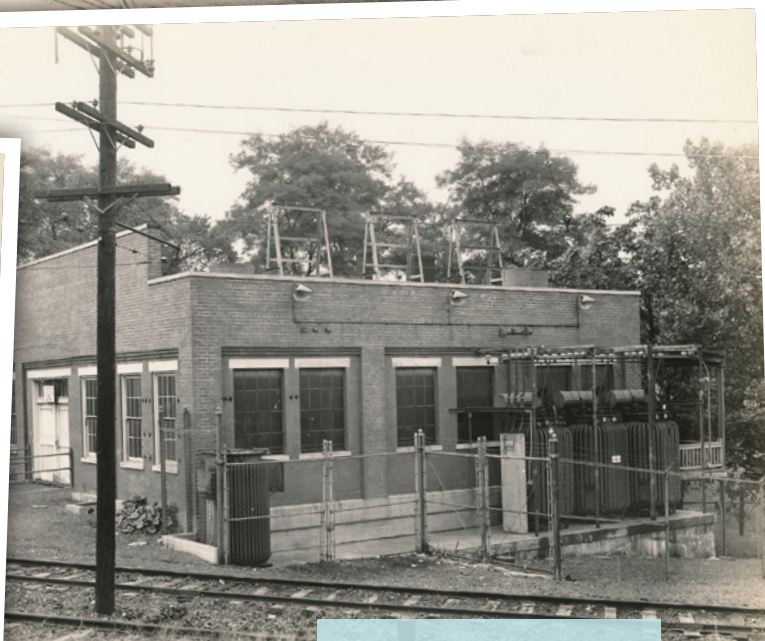
CG&E Fort Mitchell Substation, 1937
