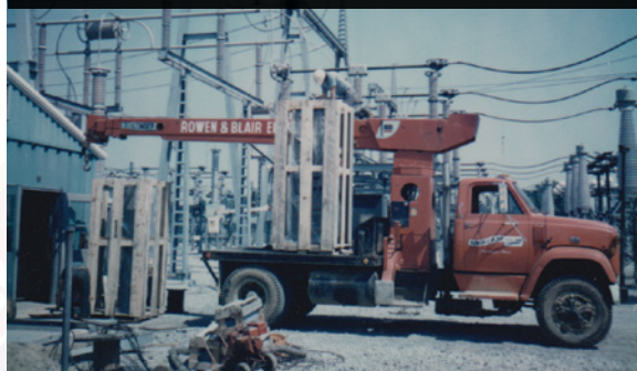
Local 131 members Ron Williams and Dick Carson at work at the Argenta substation on June 4, 1974.
