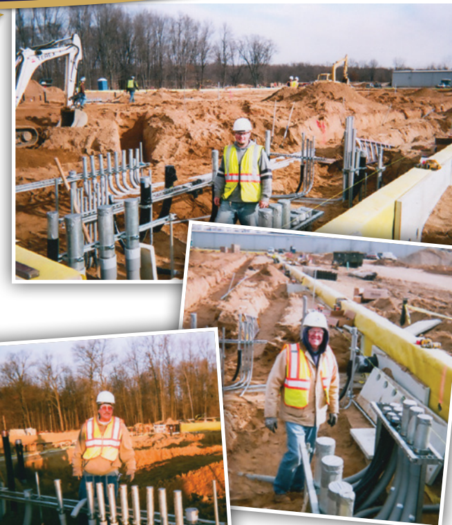
Local 131 members help build the Gun Lake Casino in 2009: (top photo) Jeff Paam, (middle photo) Mike Tiller and (bottom photo) Scott Flower.
