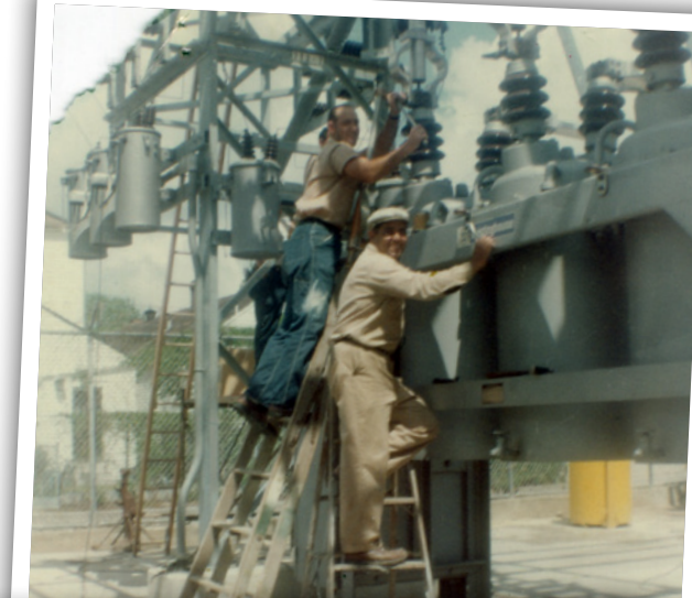
Local 130 members work on construction of the New Orleans Public Service 115,000-kilovolt electric substation at Dublin and Willow streets in 1965.
