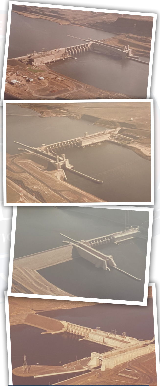
Dams built by the U.S. Army Corps of Engineers and wired by members of Local 112 for the Lower Snake River Project in southeastern Washington beginning in 1955 were (top to bottom) Ice Harbor, completed in 1961; Lower Monumental, completed in 1969; Little Goose, completed in 1970; and Lower Granite, completed in 1975.
