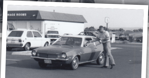
Local 112 members and other Southeastern Washington Building and Construction Trades Council members participate in an informational picket at a Buttrey Foods store in July 1981 after the company began construction of Pasco and Kennewick stores using non-union contractors from outside the area. Soon after on July 31, the council ended the picketing after Buttrey agreed to use local union contractors on its construction projects in the Tri-Cities.
