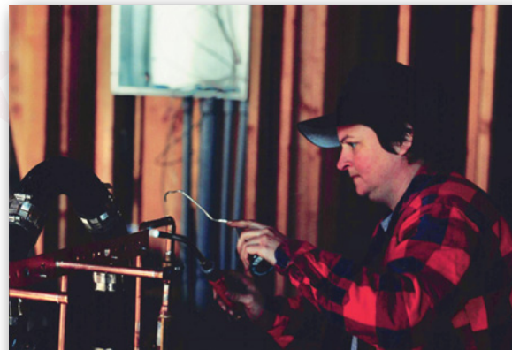
Sister Maxine Lawson of California State Pipe Trades Council-affiliated Local 342 of Concord performs plumbing work on the campus of the Shepherd's Gate women's shelter in Livermore in 1998.
