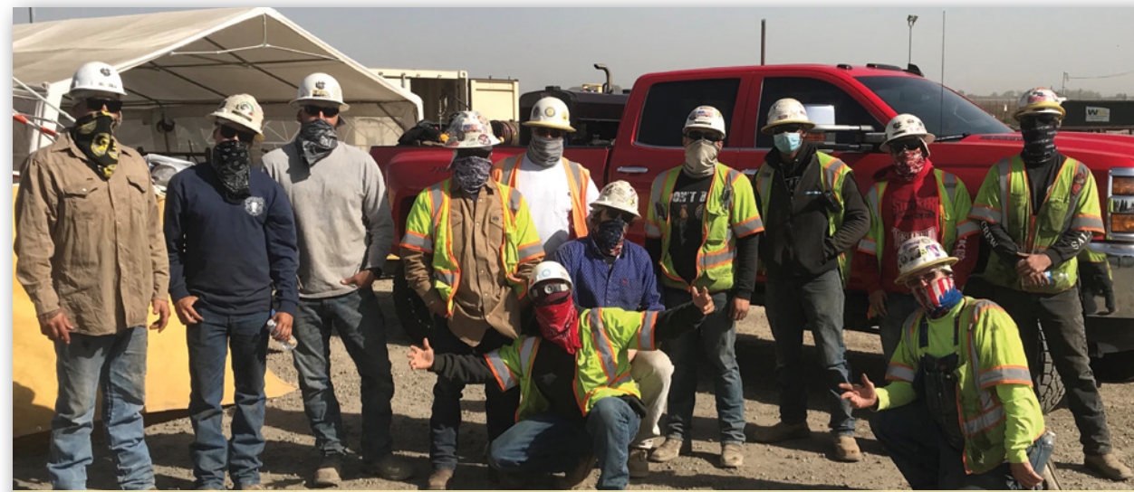
A Local 342, Concord, pipeline crew, wearing masks to protect themselves against the coronavirus (COVID-19) pandemic, works at the Pacific Gas and Electric Company (PG&E) McDonald Island gas-storage facility with Underground Construction in November 2020.
